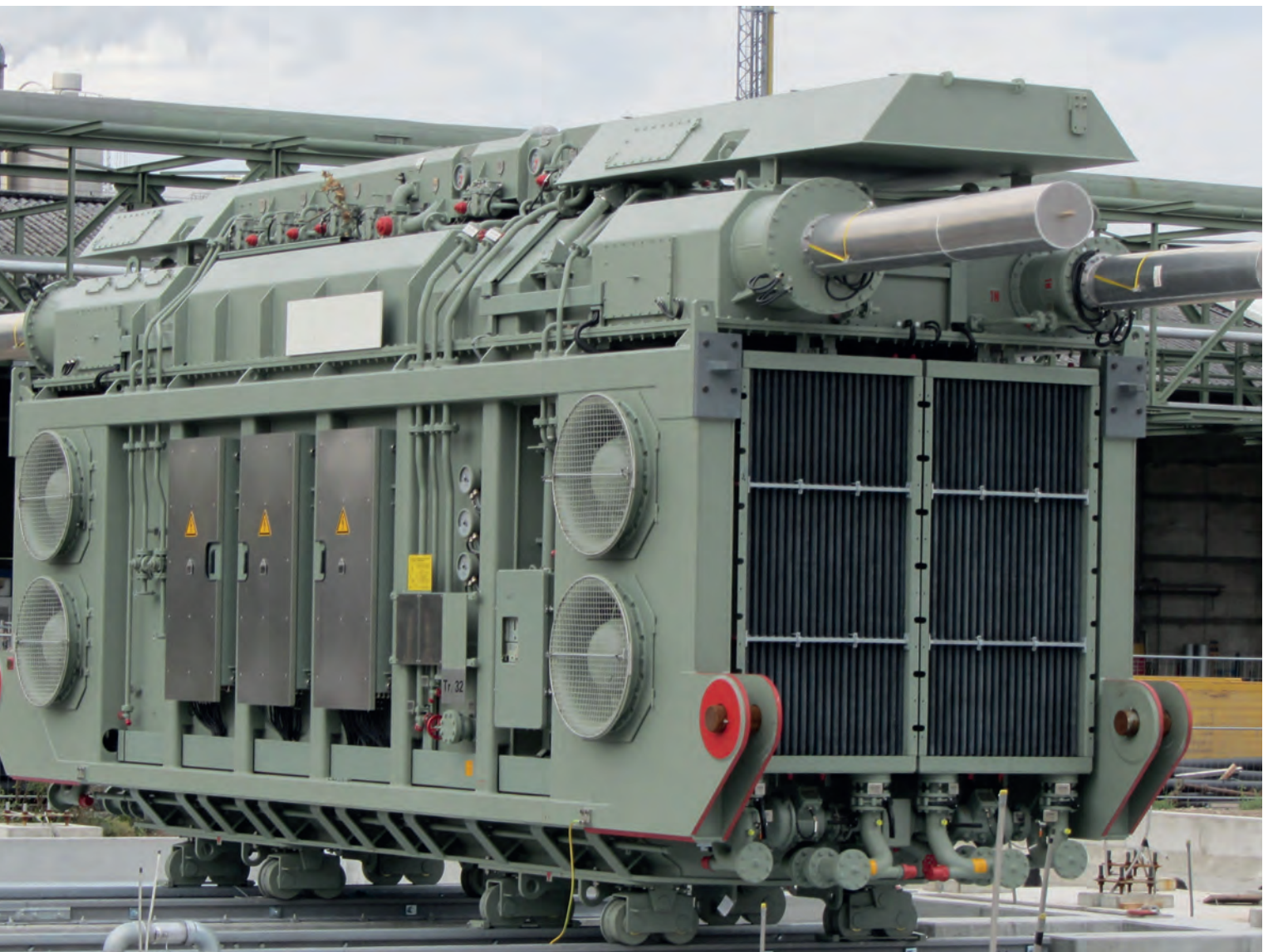
An oil-cooled power transformer supplies a chemical plant in central Germany. Provided with HEROSE valves for onshore applications.
