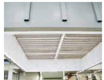
Heating elements in furnace hood
